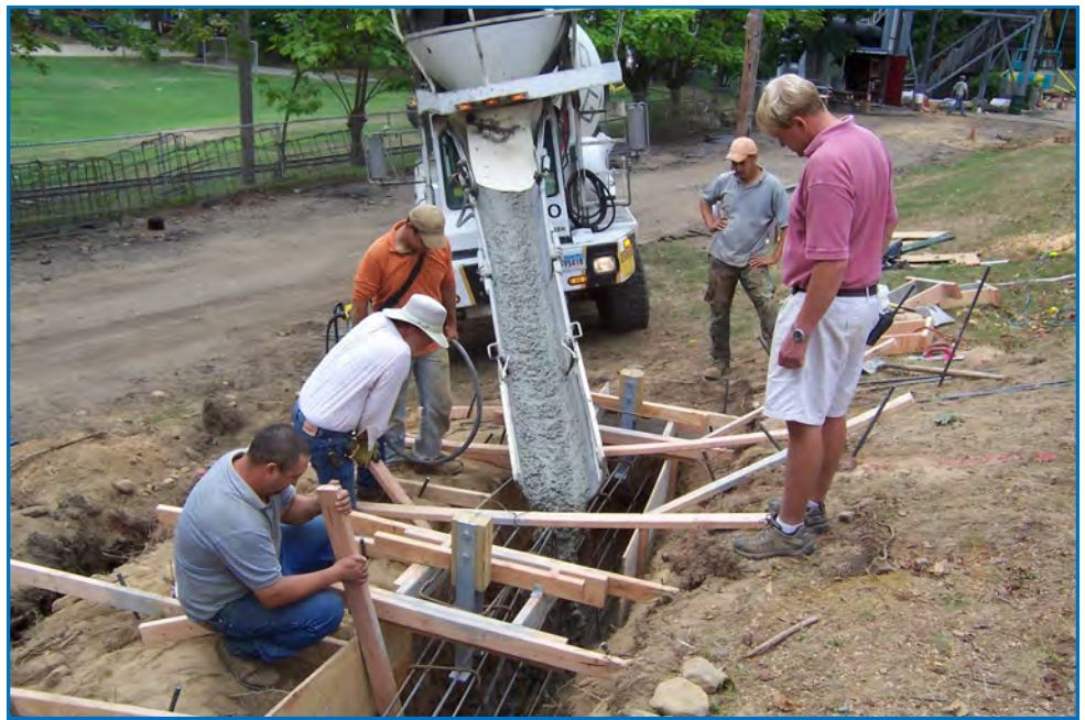
Quassy's Eric Anderson (right) watches as concrete footings are poured during the late summer of 2010 for the park's new roller coaster.
